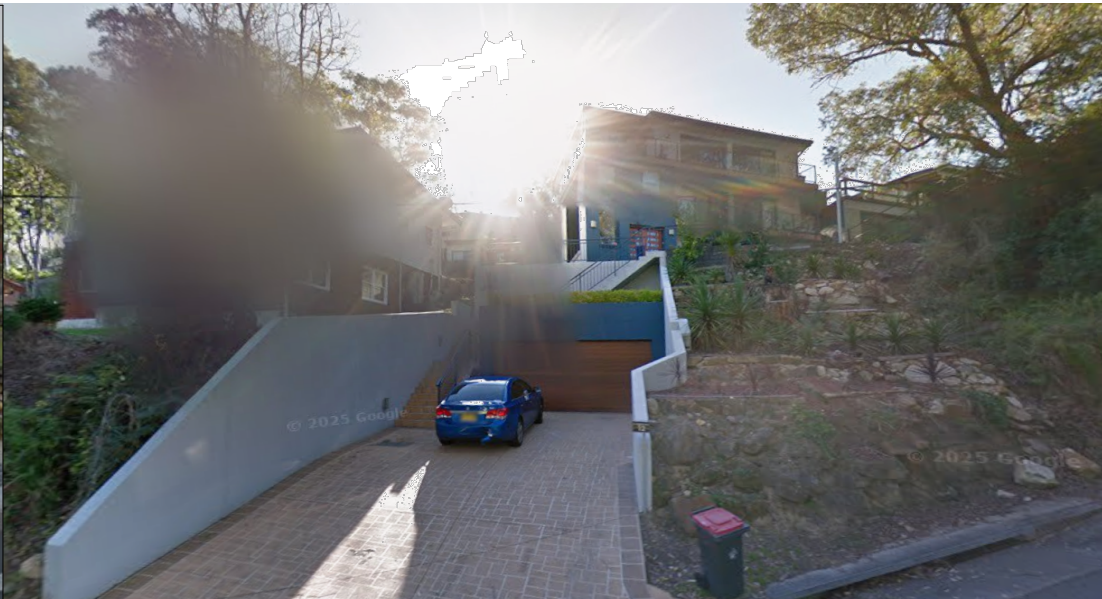
NO.12 CARINYA ROAD PICNIC POINT - 3 STOREY SINGLE DWELLING
