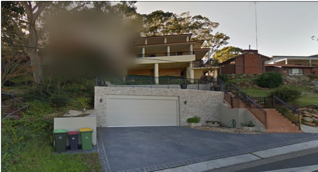
NO.18 CARINYA ROAD PICNIC POINT - 4 STOREY SINGLE DWELLING
